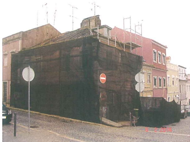
Travessa Paulo Martins, 11-15 – obra
